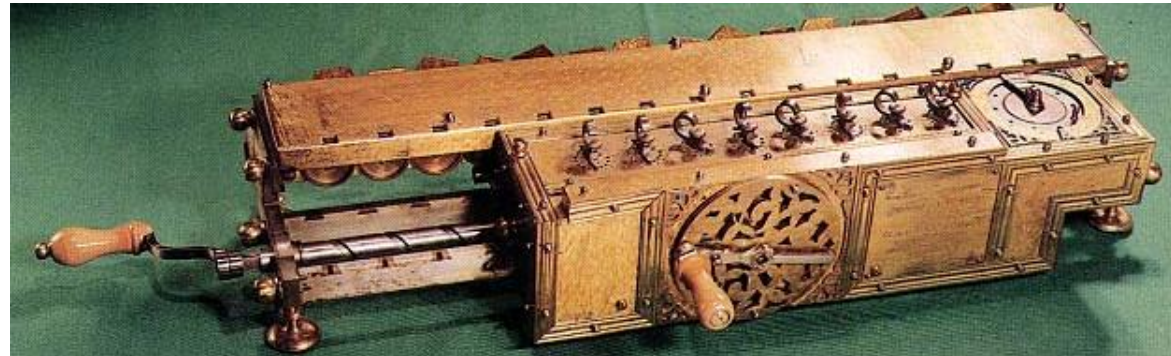
1673: 4-function mechanical calculator (addition, subtractions, multiplication, division)
